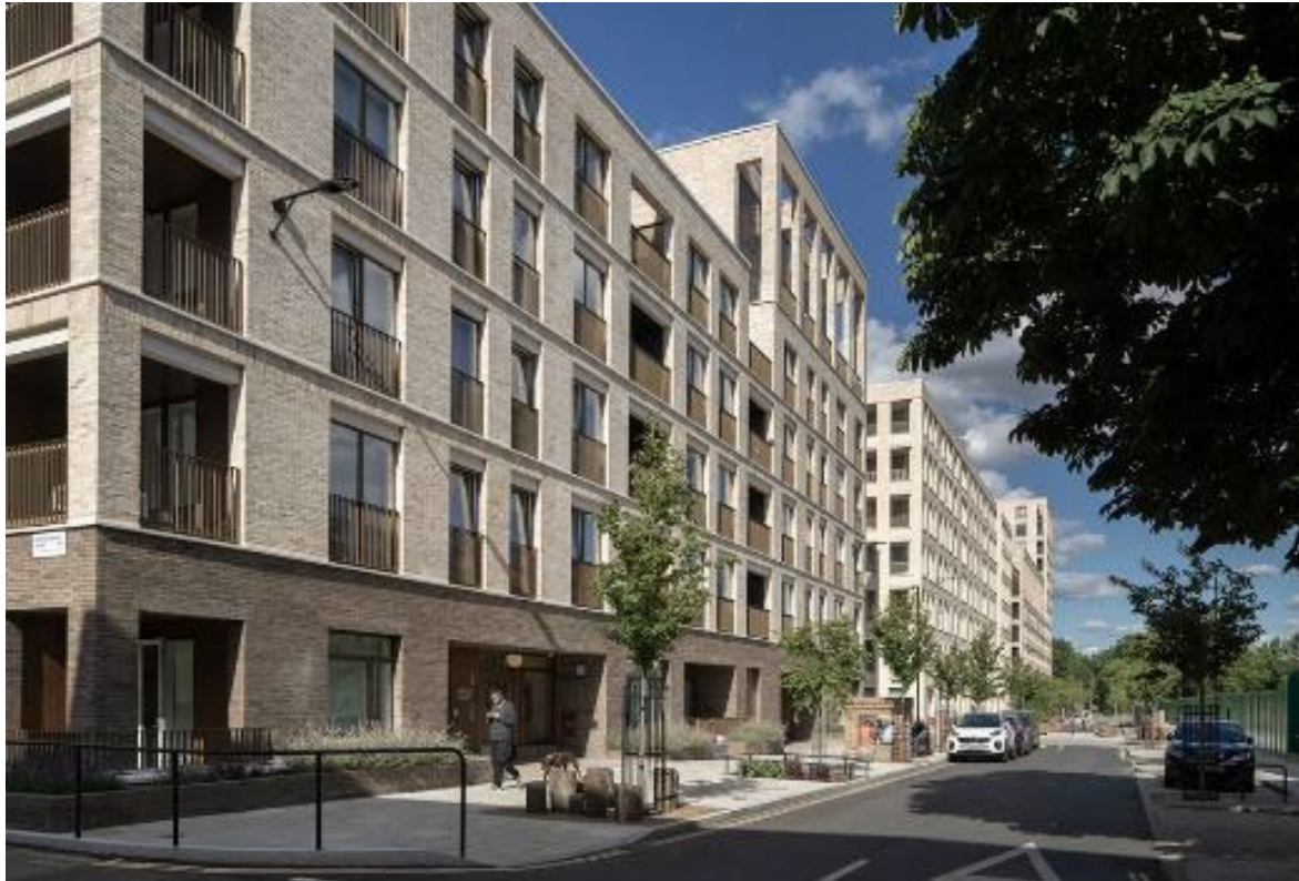
Figure 83 – Kings Crescent Estate Phases 1 & 2, Hackney: A local authority-led development involving intensive consultation with residents and local people who helped to define all aspects of the scheme including the planning of streets, internal layouts and material specifications. Three courtyard buildings combine existing and new blocks with shared amenity spaces and dual aspect entrance lobbies featuring the same level of design quality regardless of tenure.
