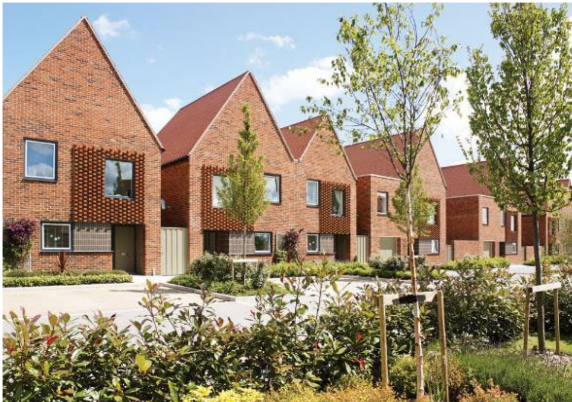
Figure 38 – Horsted Park, Chatham: Pairs of semi-detached houses with recessed entrances and expressed gables provide a strong rhythm to the streetscape. Projecting chequerboard brickwork patterning provides a visual identity and sense of character.
