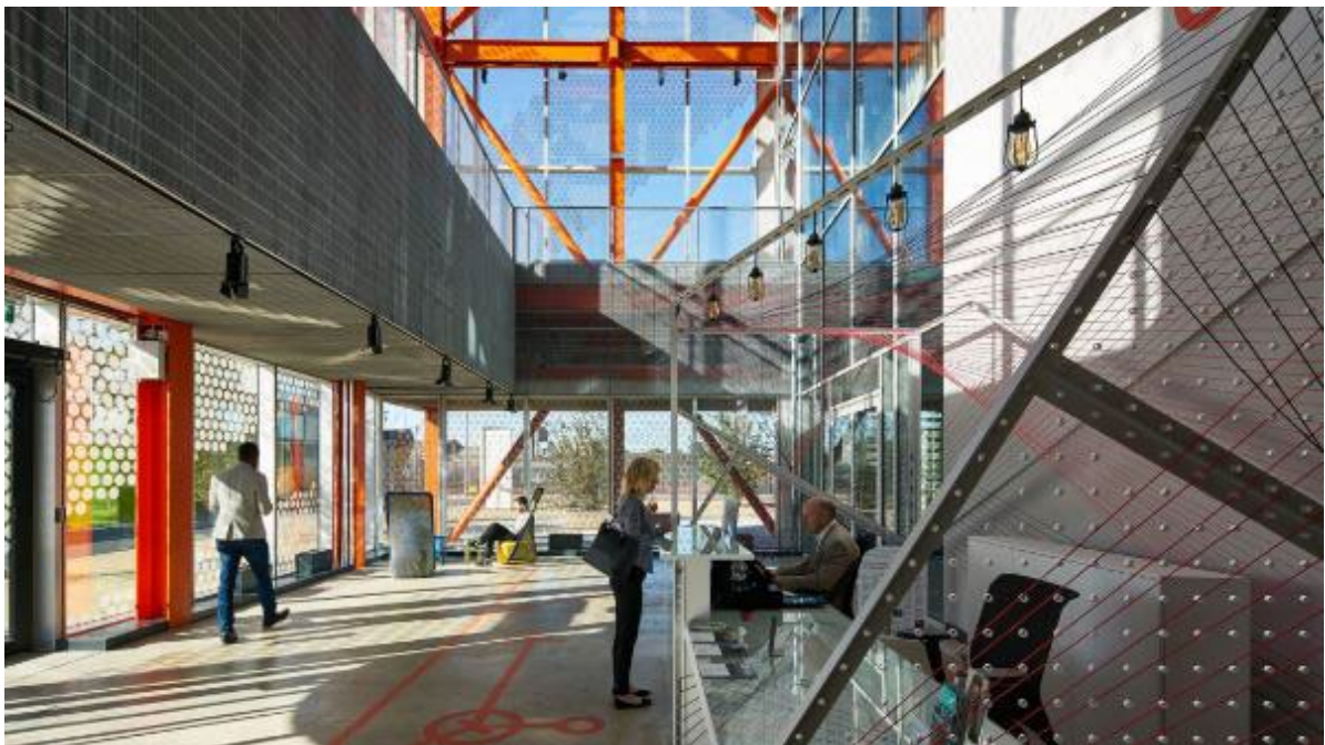
Figure 49 – Here East, Stratford: The refit of the London 2012 Media Centre into commercial space for creative and digital industries was inspired by the light industrial factories and yards of neighbouring Hackney Wick. The aim was to make a series of huge buildings more social, dynamic and flexible with the potential to evolve. The original windowless facade was removed to create a glazed outer layer of flexible work, studio and commercial spaces around the perimeter - maximising natural daylight, ventilation and views. Education, employment and enterprise coexist behind colourful animated facades featuring projecting/inset balconies with bright orange metalwork, brise soleil, and solar dot patterned glazing. The combination of elements is effective in breaking down the scale of the building.
