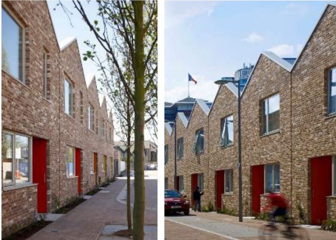
Figure 39 – Anne Mews, Barking: Traditional terraced houses focusing on the simple application of high quality materials and a generosity of scale, featuring large window openings, recessed entrances and integrated bin storage. The scheme creates a strong street frontage and a welcoming streetscape.
