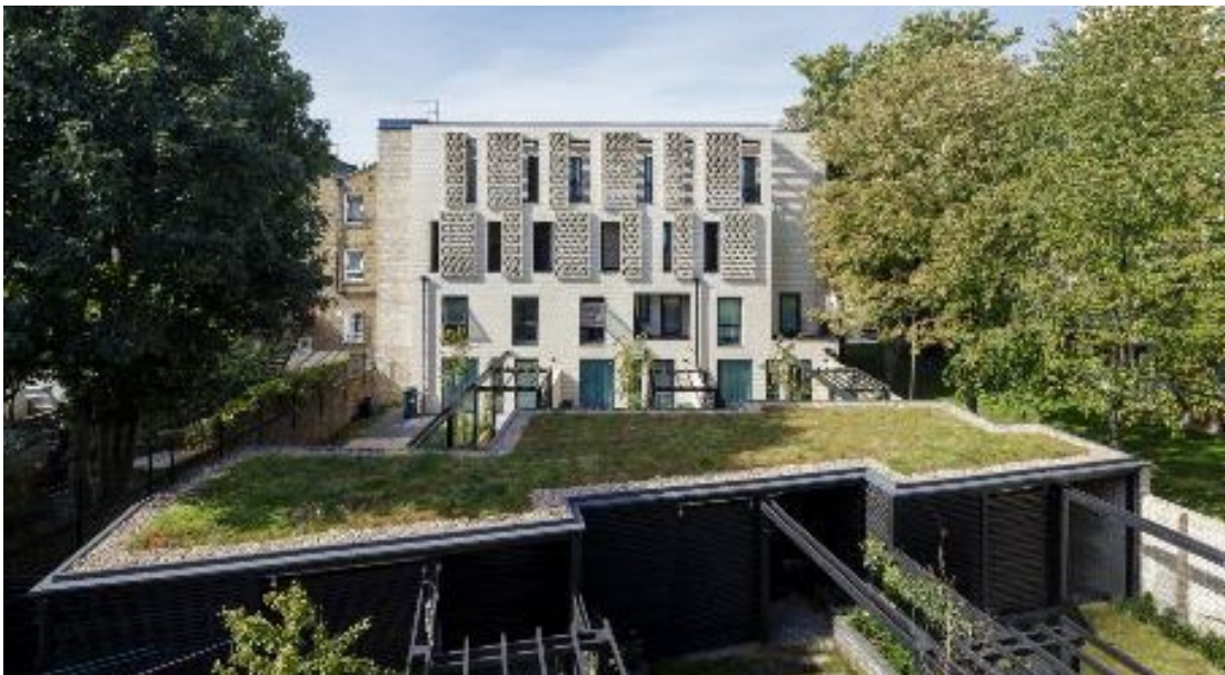
Figure 43 – Vaudeville Court, Islington: The design features a mix of maisonettes on the ground and first floors, and two-bedroom flats above. Arranged in two terraces, with private gardens between them, the scheme references the scale of neighbouring buildings and reinstates the street frontage. The family homes are dual aspect with open plan living space and a private courtyard garden. Garden rooms give families extra amenity and storage space.
