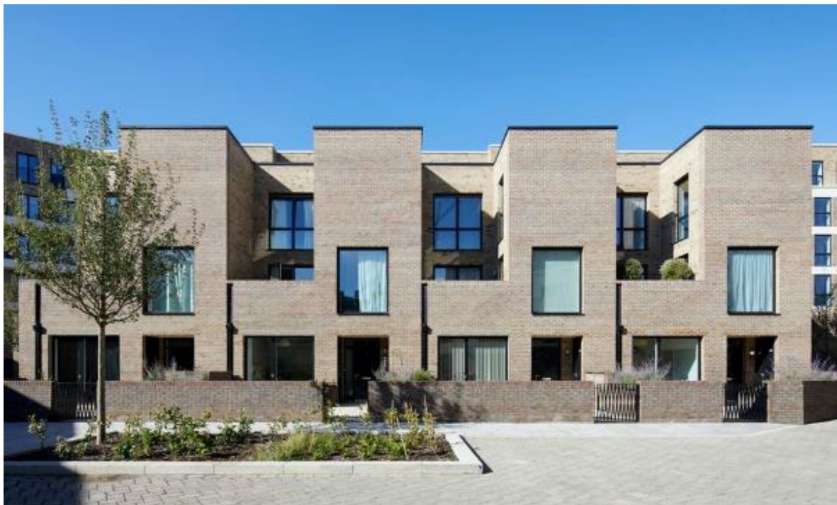
Figure 31 – Park View Mansions, Chobham Manor: Generously sized openings help to break up the mass of the three-storey townhouses, the positioning adds rhythm to the facade animating the elevation.
