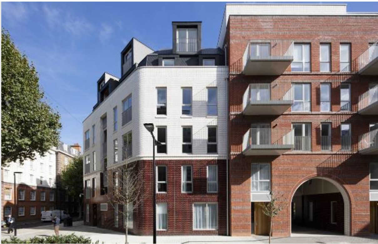
Figure 8 – The Bourne Estate, Camden: A sensitive contextual approach introduces two new blocks within an existing Grade II listed estate to complete the original layout. The buildings respond to the form and scale of the original architecture with fine brick detailing and a high-quality finish.
