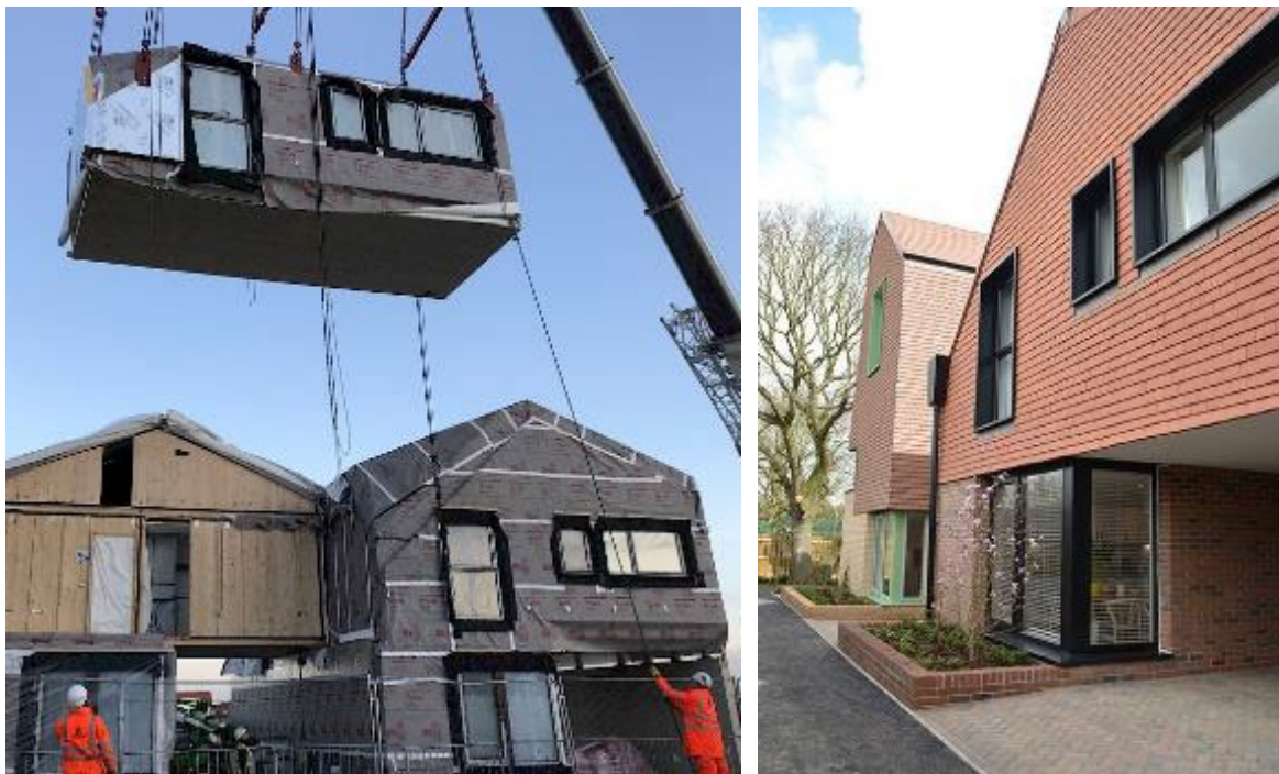
Figure 92 – Beechwood West, Basildon: A new neighbourhood of over 250 volumetric family houses utilising factory-built modular technology offering a choice of housing typologies, layouts and external finishes, precision engineered in an efficient and sustainable way with a significant reduction in construction waste compared with traditional build methods.
