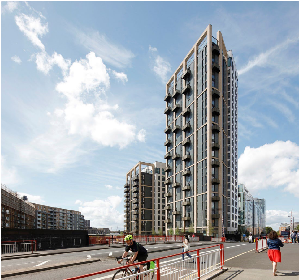
Figure 93 – Union Wharf, Greenwich: One of the first high-rise residential projects in the UK to use volumetric off-site construction; although initially designed to be delivered traditionally, the rationalisation of design elements and a repeated floorplate enabled its conversion to modular build construction, retaining design quality while maximising the benefits of off-site design and delivery.
