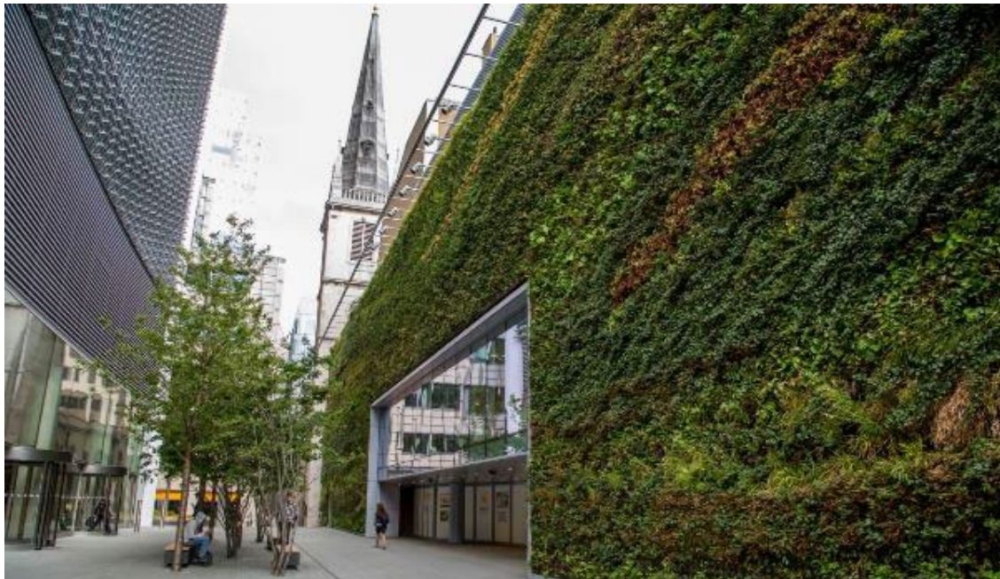
Figure 96 – Fenchurch Street, London: At over 700sqm this living wall contains around 52,000 plants. The wall was installed on an annex service building opposite the southern entrance providing visual amenity with urban climate mitigation and biodiversity benefits.
