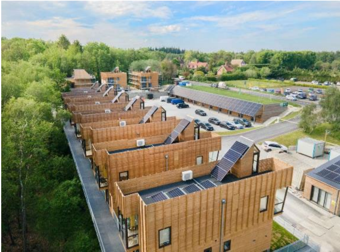
Figure 46 – Flimwell Park, East Sussex: A sustainable mixed-use development in a rural setting comprising of a mix of uses including workspace, education, residential, restaurant and amenities. Environmental, social and economic sustainability were at the heart of the project.
