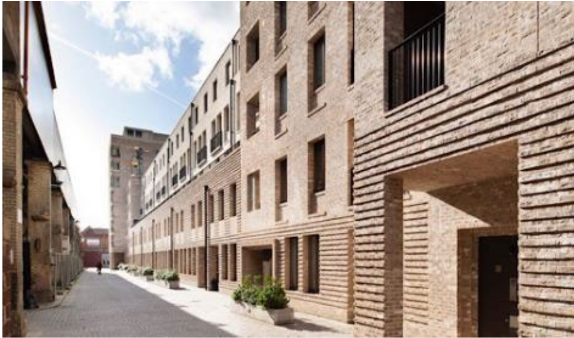
Figure 41 – Silchester Estate, Kensington and Chelsea: A mix of housing typologies combined to create a legible human scale urban block enclosing a shared garden. Openings have a vertical emphasis with regular repeated proportions creating a rhythm to the streetscene. All homes are dual aspect providing good levels of daylight and cross-ventilation with access to private amenity space.
