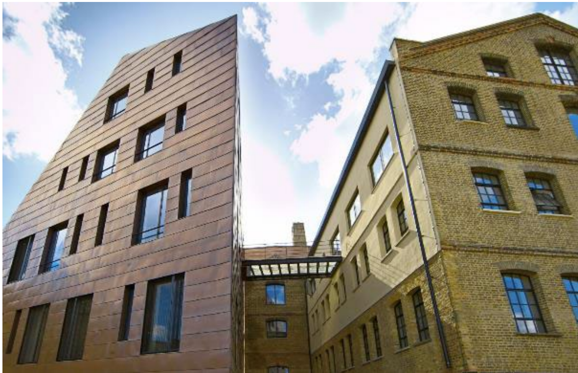
Figure 30 – The Granary, Barking: A new bronze clad extension takes its cue from the gabled form of the original building and is attached via the vertical circulation core and a high level bridge link. The contemporary design clearly distinguishes the 'old' from the 'new' whilst respecting the existing 19th Century building.
