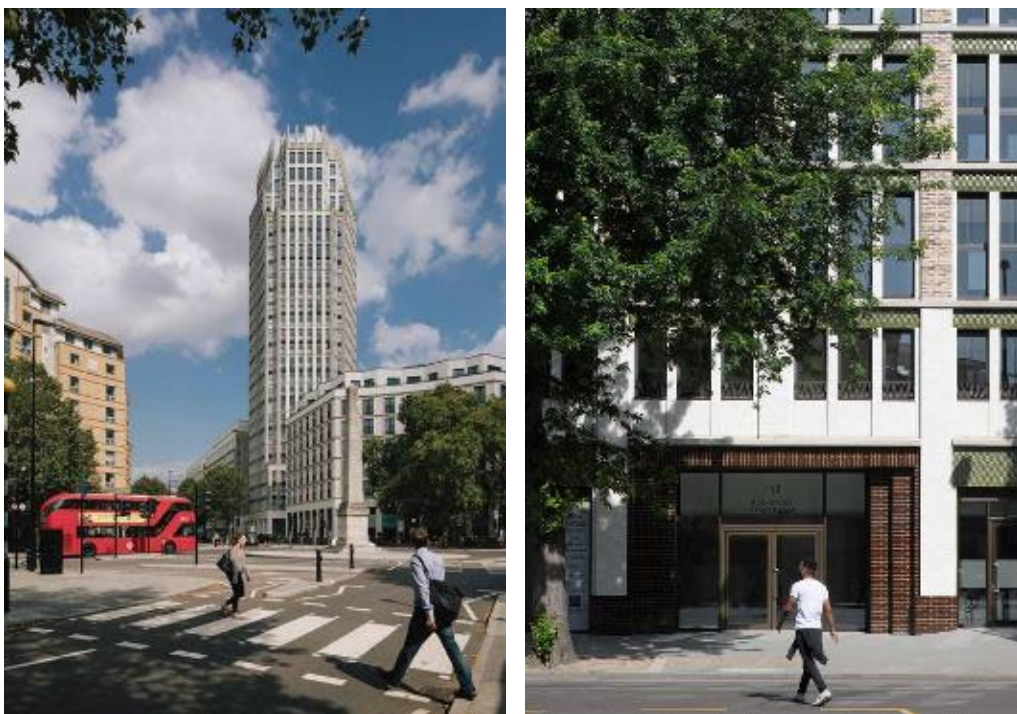
Figure 19 – Blackfriars Circus, London: Introduces a 28-storey tower with a slender facade and pre-cast sills at every other level to create a strong vertical emphasis, a variety of stock and glazed bricks are used to enhance key elements of the building including a colonnaded base. The selection and application of materials helps to differentiate and establish a unique identity.
