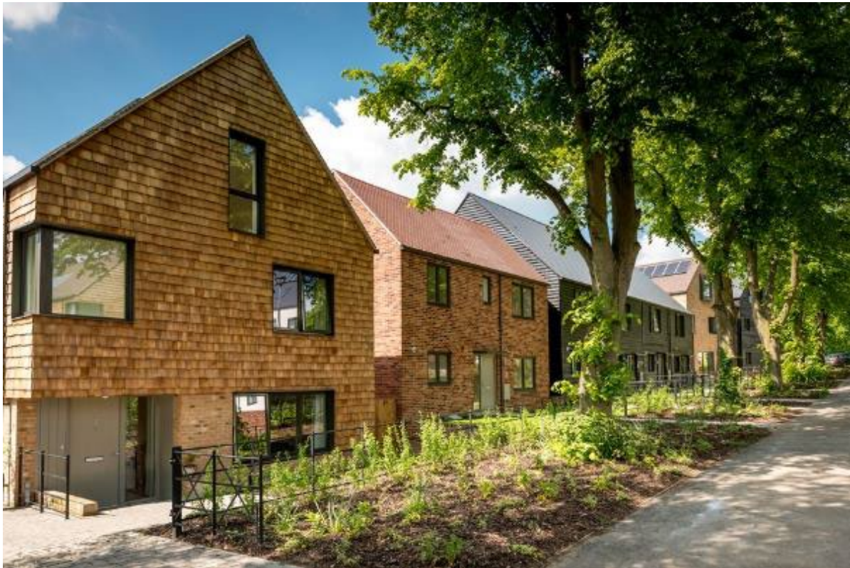
Figure 28 – The Avenue, Saffron Walden: Sympathetically designed to reflect the character of the surrounding area with a mixed palette of materials and crisp contemporary design detailing.
