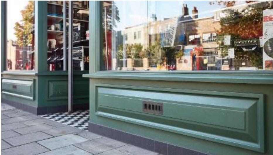
Figure 56 – A traditional shopfront stallriser
