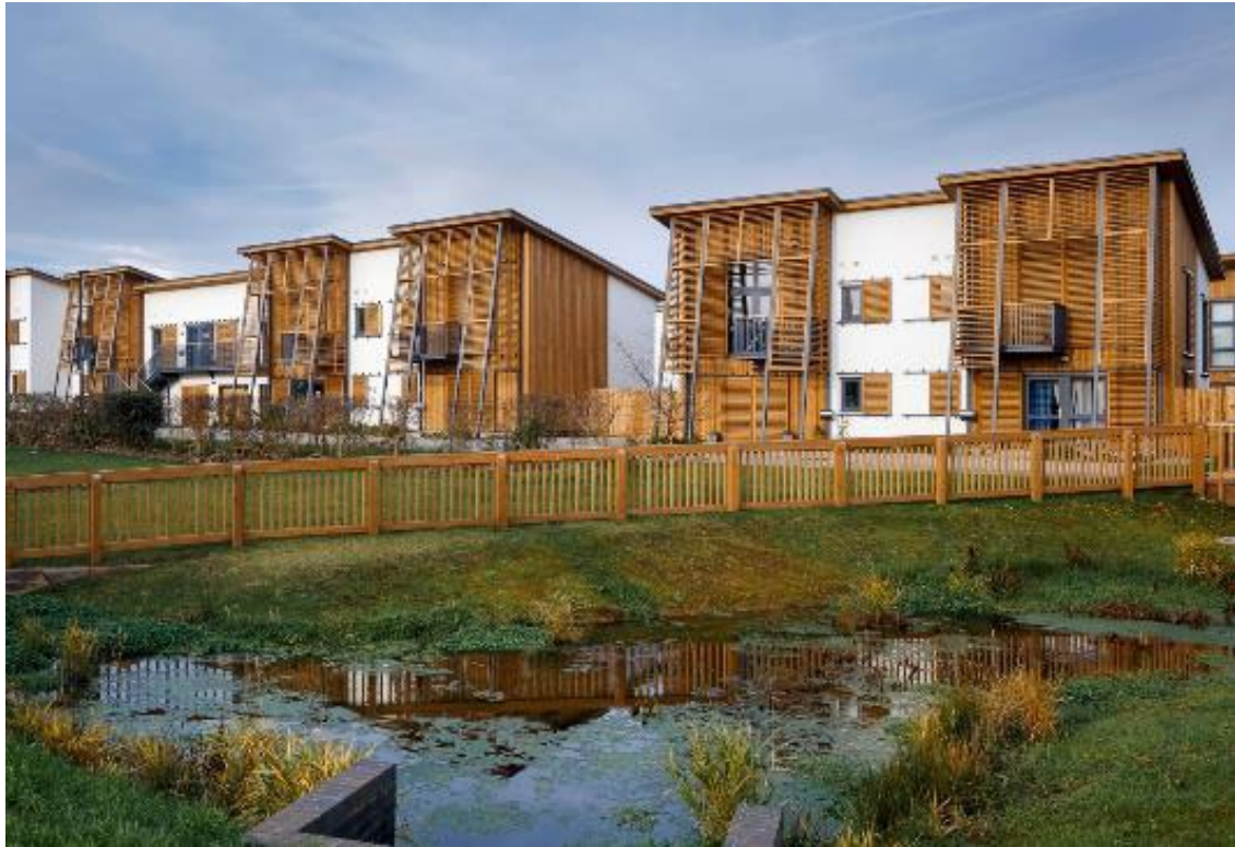
Figure 91 – Hanham Hall, South Gloucestershire: 187 homes built from factory made elements which minimise waste and are energy efficient to produce and build, the zero-carbon standard is achieved by using an efficient building envelope constructed using Structural Insulated Panels (SIPs) and roof-mounted PVs. The homes combine stack and cross ventilation, large openings, deep roof overhangs, balconies and shutters to avoid overheating.
