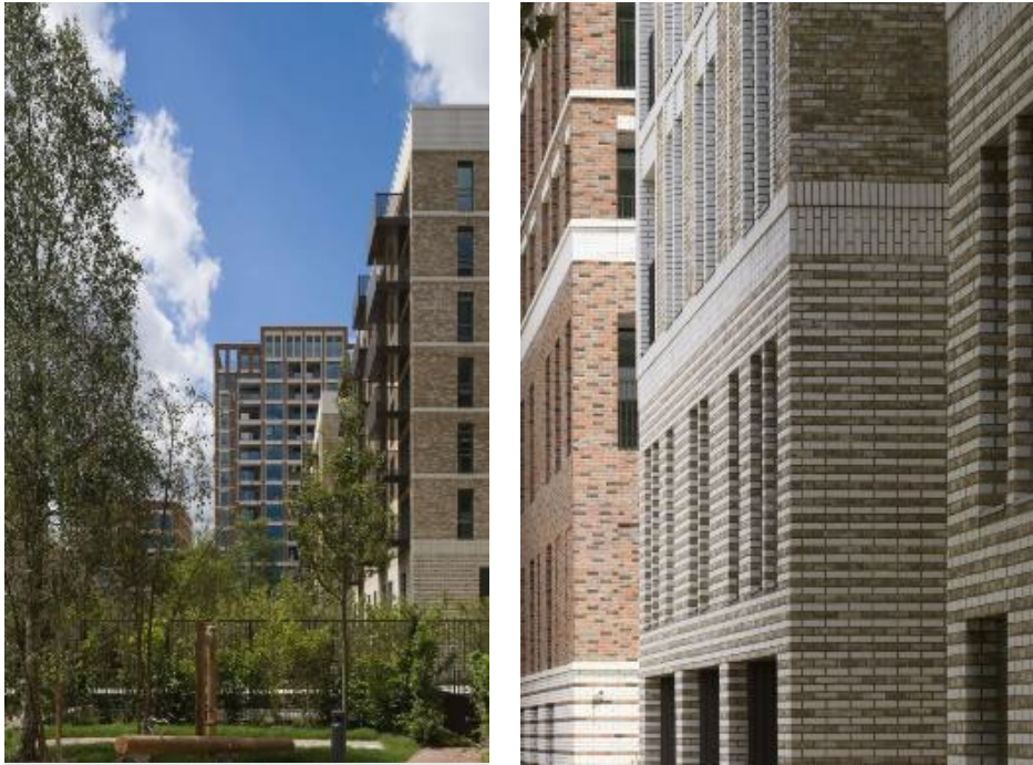
Figure 18 – Elephant Park, London: Creates a distinctive neighbourhood comprising of townhouses, mansion blocks and a 16-storey tower; executed in blends of five different bricks creating a playful, decorative effect which breaks down the volume of the large-scale blocks.
