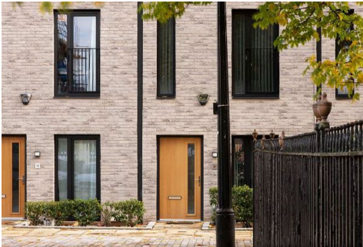
Figure 29 – Timekeepers Square, Salford: A limited materials palette is used throughout the scheme; predominantly a light brick in response to the sandstone of the nearby Grade II listed church. The materiality and architectural detailing is simple and restrained.
