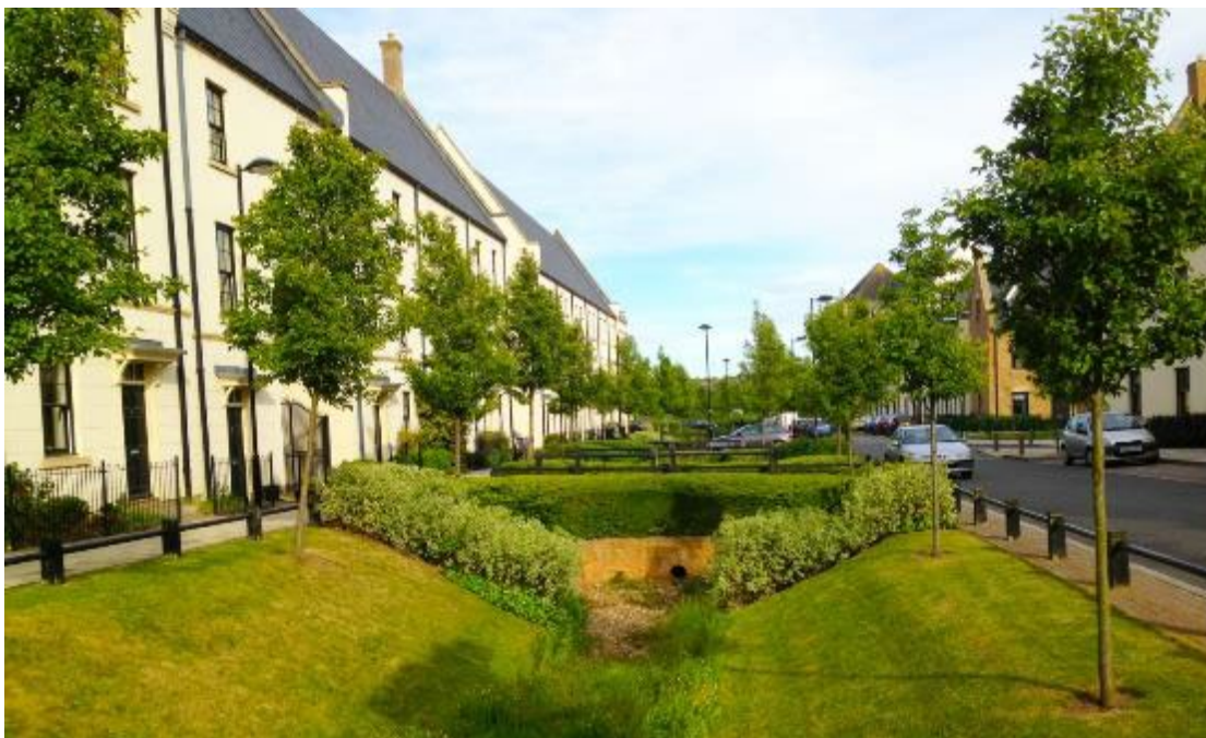
Figure 95 – Upton, Northampton: Sustainable Urban Drainage Systems are incorporated throughout the masterplan (an urban extension of approximately 1350 homes) with generously sized swales contributing to the character, identity and biodiversity of the neighbourhood. The swales have both functional and aesthetic benefits; reducing flood risk by storing and infiltrating water runoff, whilst also creating attractive green corridors which soften the streets.
