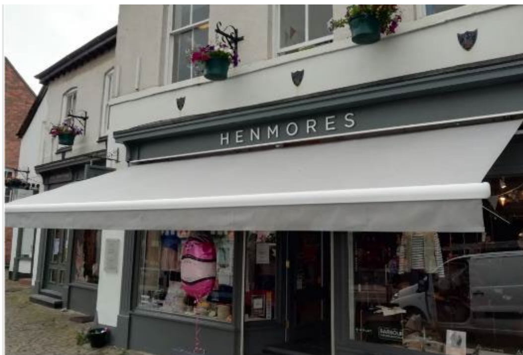
Figure 60 – A fully integrated retractable canvas canopy
