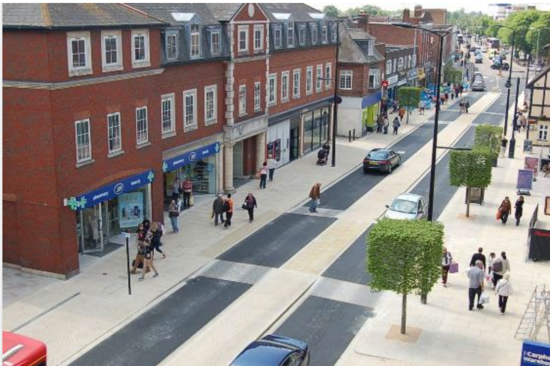
Figure 80 – Hornchurch Town Centre, Havering: A key feature of the scheme was a focus on improving pedestrian permeability. This was achieved by removing guardrails, placing crossings on desire lines, increasing the width of the footways and implementing a continual central pedestrian crossing strip. The scheme also improved social spaces through planting, new lighting, wayfinding and street furniture. Traffic flow was also improved, bus stops were made fully accessible, and better provision for cycling was installed.
