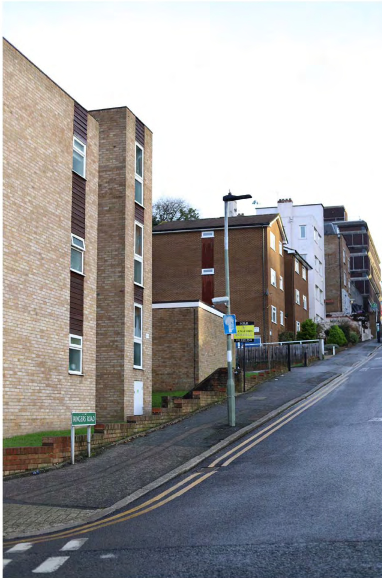
Description: View from Ravensbourne Road, looking north-east along Ringers Road to Bromley High Street.
