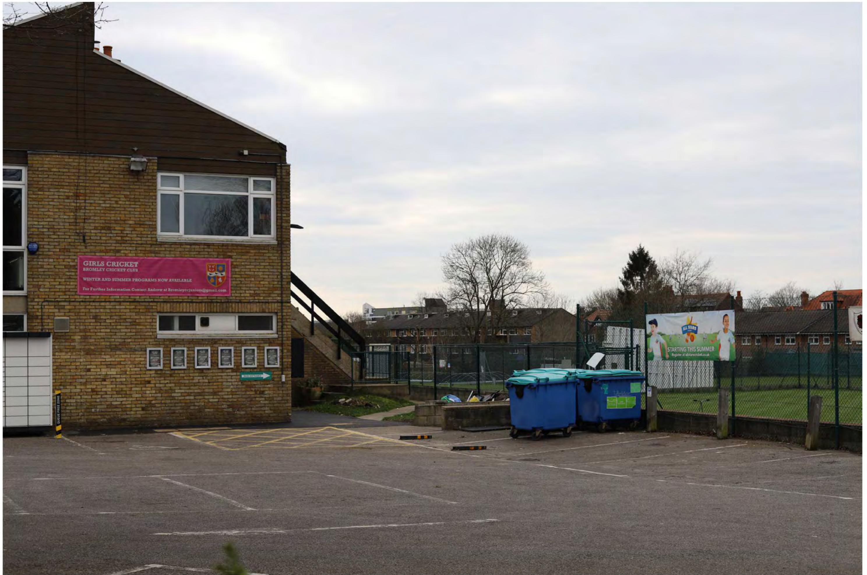
Description: View from Plaistow Lane, looking south-west towards Bromley Town Centre.
