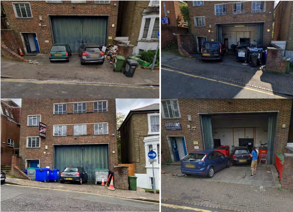
Figure 1: Ethelbert Road Parking Spaces
