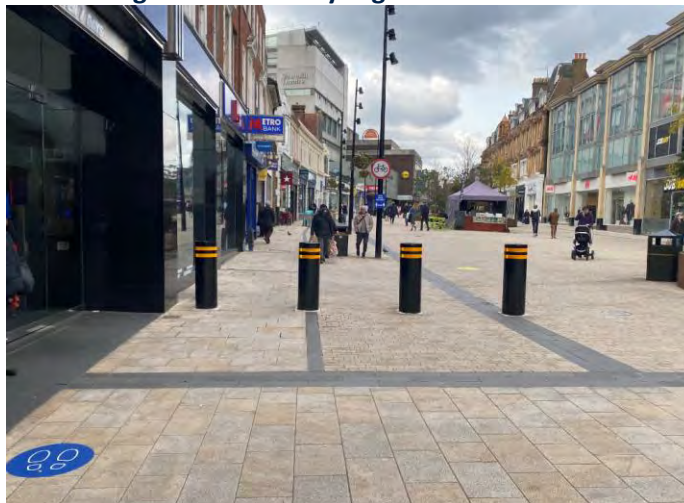
Figure 4 – Bromley High Street
