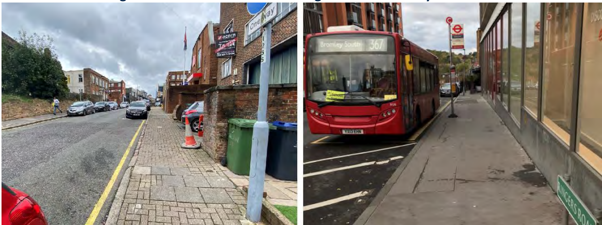
Figure 2 – Ethelbert Road and Ringers Road Footways
