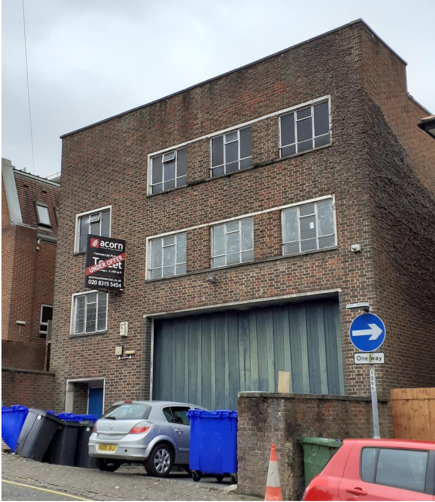
Photo 3. B2 block of flats facing Ethelbert Road.
