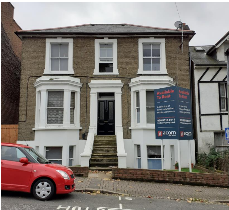
Photo 2. Building B1 from Ethelbert Road.
