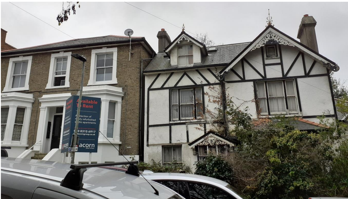
Photo 5. Old uninhabited house with overgrown garden directly next to building B1.
