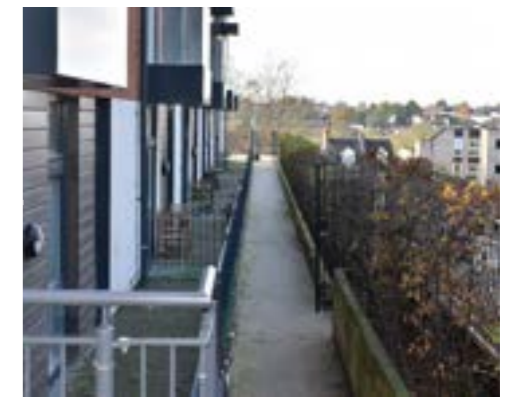
Planters with Hedgerow along the frontage of a recent residential scheme, providing privacy as well as a soft frontage of the building
