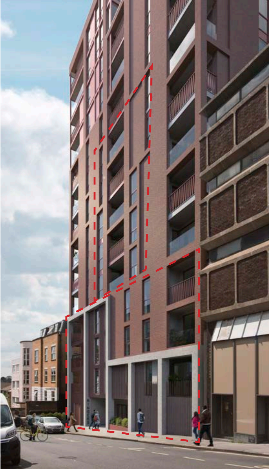
Street level plinth with vertical metal louvres to base of Block A
