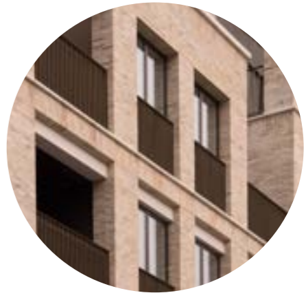
Vertical brick feature banding
