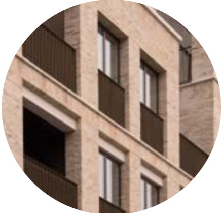
Vertical brick feature banding
