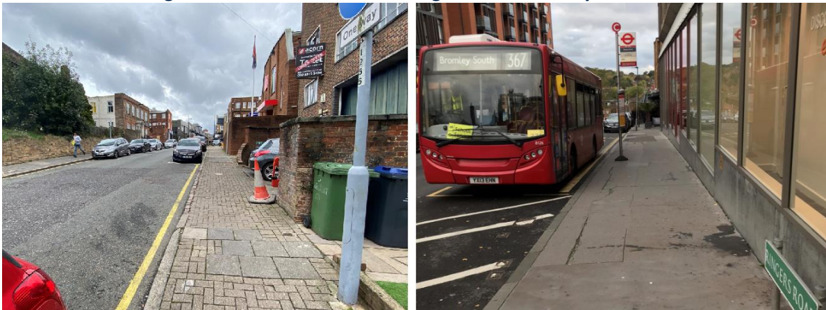
Figure 6 – Ethelbert Road and Ringers Road Footways
