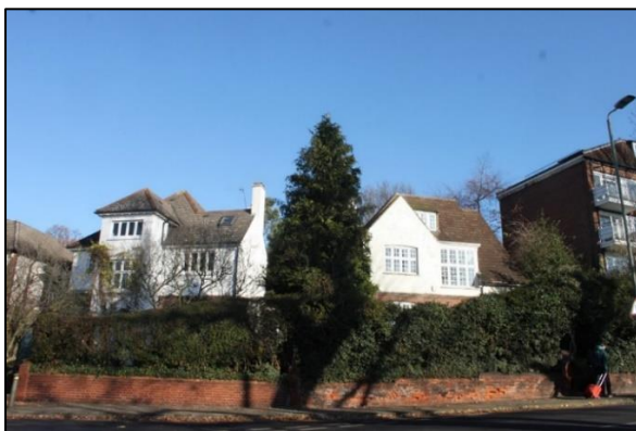
Fig. 24. 2 Farnaby Road and 14 Beckenham Lane, west elevations
