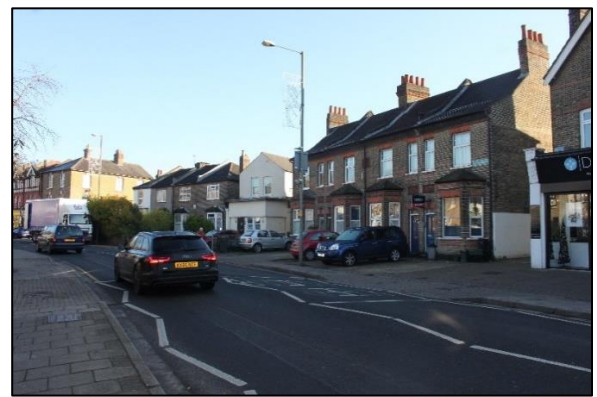
Fig. 27. 57 to 73 Beckenham Lane, north elevations
