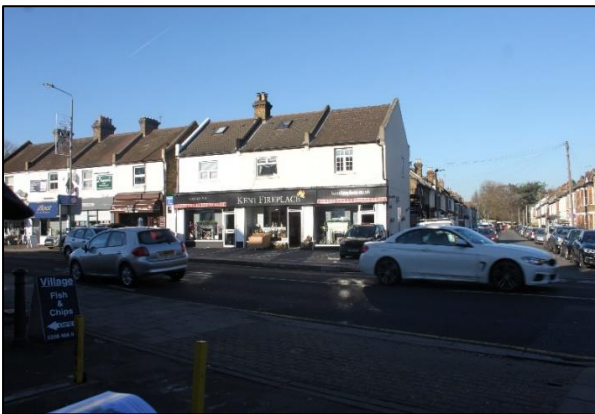
Fig. 35. 96 to 108 Beckenham Lane, south elevation
