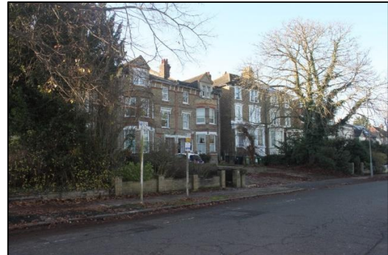
Fig. 19. 46 to 50 Valley Road, east elevations
