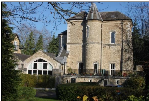
Fig 17. Old Pumping Station, west elevation
