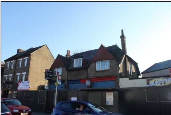
Fig. 29. Valley Coffee House, north and west elevation, now boarded up
