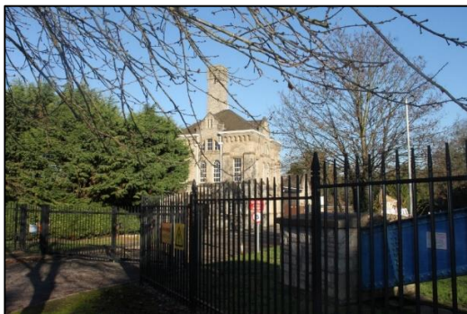
Fig. 18. Main Pumping Station, west elevation
