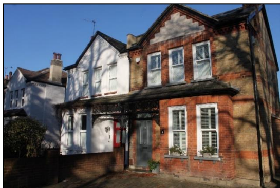
Fig. 54. 8 and 10 Ravensbourne Avenue, west elevation
