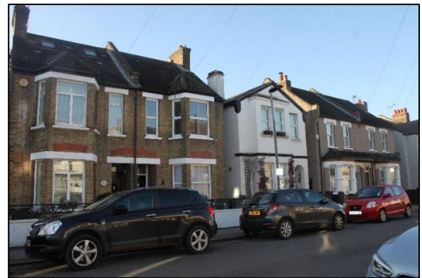
Fig. 50. 15 to 23 Meadow Road, west elevations
