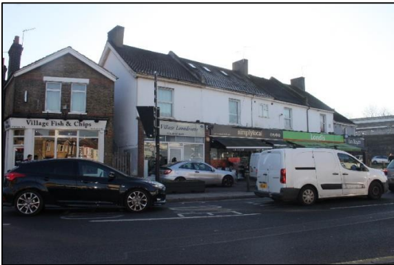
Fig. 30. 89 to 99 Beckenham Lane, north elevations
