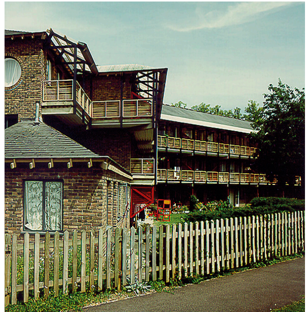
Figure 24: In this housing association scheme, solar shading is provided by balconies and overhangs
