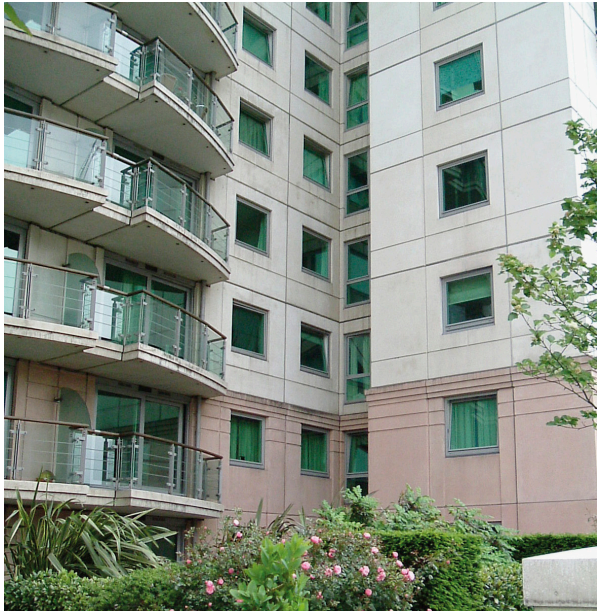
Figure 6: Windows near internal corners, such as the corners of courtyards, are usually heavily obstructed
