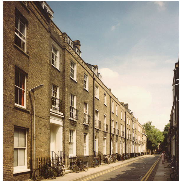
Figure 3: In Georgian streets the small spacing-to-height ratio is compensated for by tall windows. Note how window head height increases for the lower floors which are more heavily obstructed.
