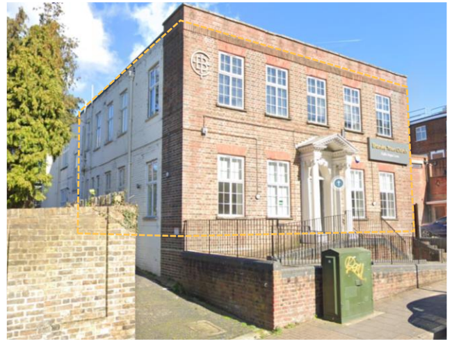
Figure 26: 2 Ethelbert Road windows.
