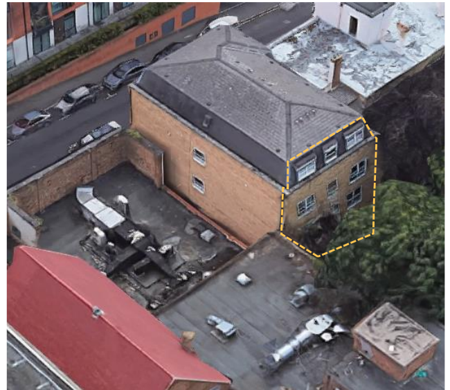
Figure 12: Simpsons Place windows.
