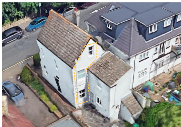
Figure 28: 11 Ethelbert Road windows.
