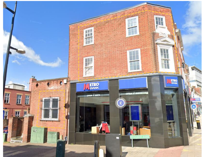
Figure 32: 72-76 High Street windows.
