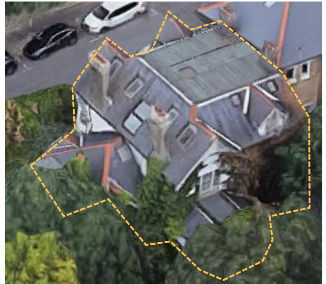
Figure 22: 7 Ethelbert Court windows.
