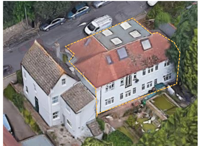
Figure 24: 1 Ethelbert Court windows.
