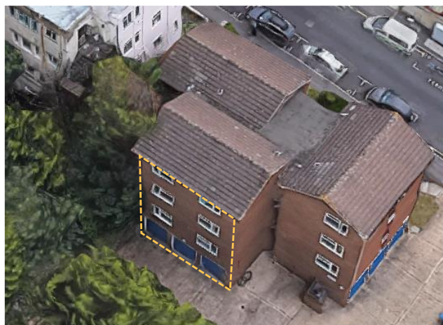
Figure 16: Harestone Court windows.
