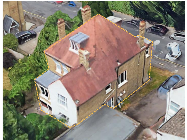
Figure 30: 13 Ethelbert Road windows.
