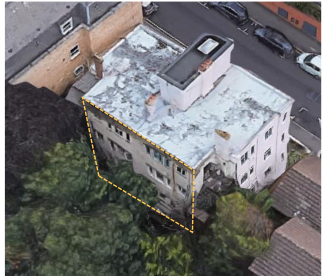
Figure 14: Ringers Court windows.
