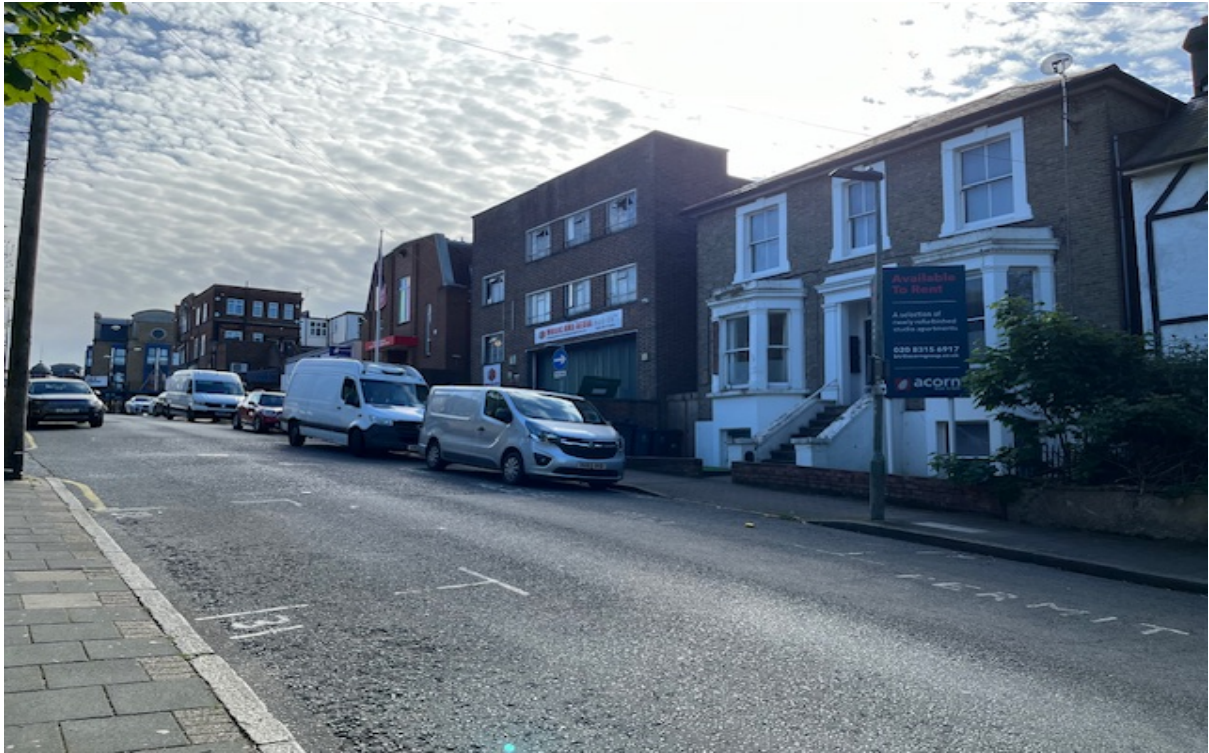
Ethelbert Road: Salvation Army building, site frontage
