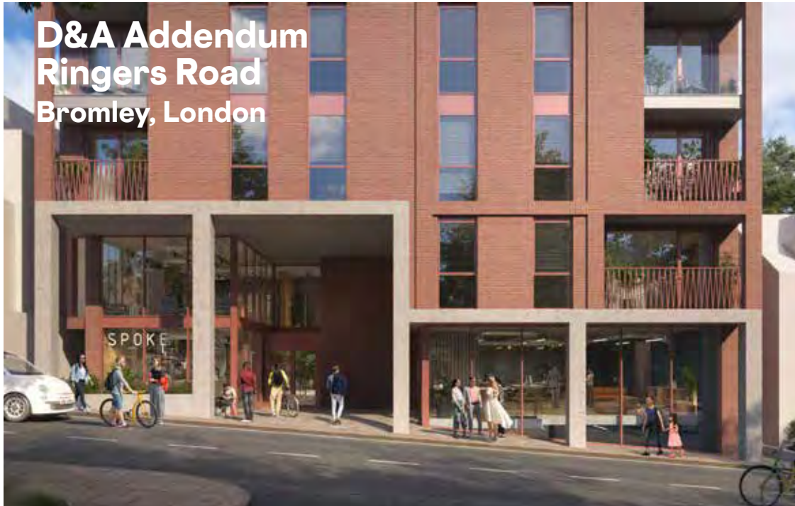
Fig. 4.15 The rendered image on the front cover of the DAS Addendum showing the limited public space made available on the Ethelbert Rd frontage, almost none of this is green. Two people are shown standing in the parking area as the narrow footpath leaves little room for social space.
