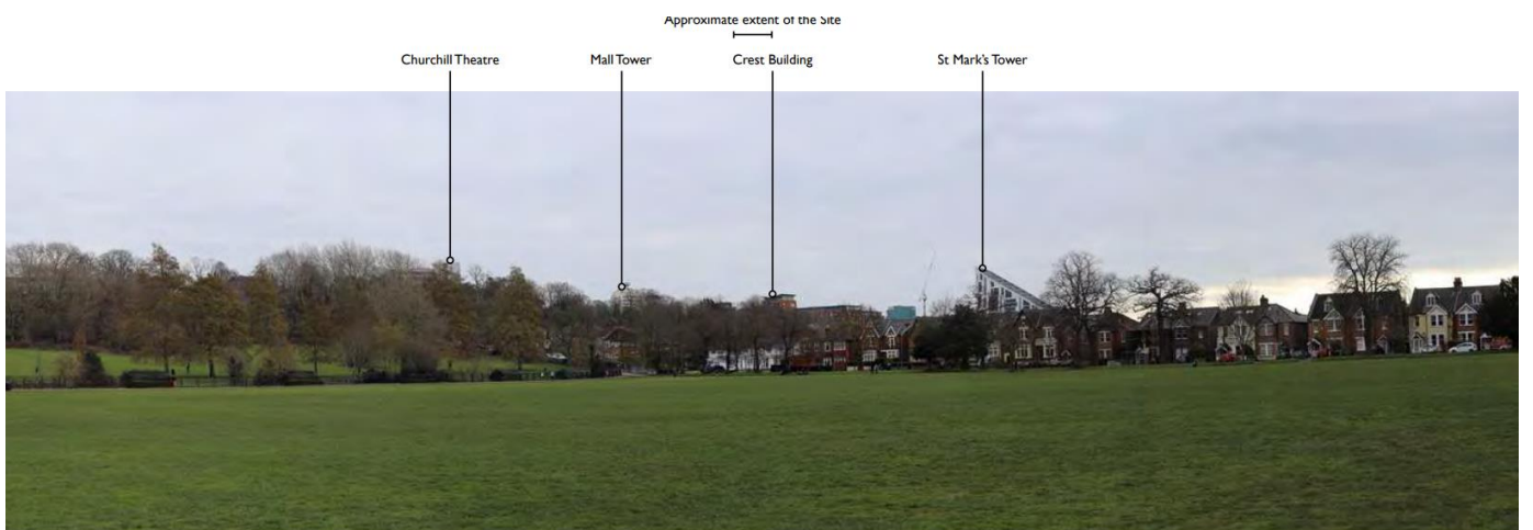
Figure 9: Viewpoint 17 (within the Conservation Area): TVIA, Part 4 looking east from Queen's Mead illustrating the open setting to the west of the hill-top town centre with its suburban fringe and with isolated taller buildings breaking the skyline.
