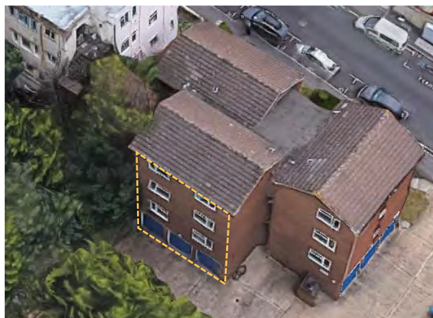
Figure 16: Harestone Court windows.
