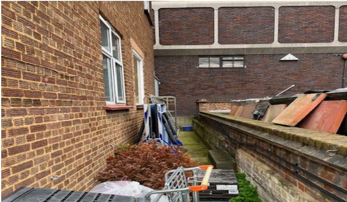
View standing south eastern corner of SA grounds parallel with rear elevation looking east toward rear elevation of No.64 TK Maxx (appeal site boundary to south) right of photo
