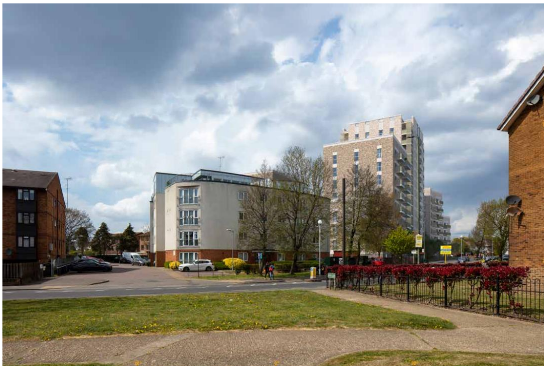
Figure 13: Proposed View from Burnt Ash Lane at Ryder Close (Source: Heritage, Townscape and Visual Impact Assessment (Feb, 22))
