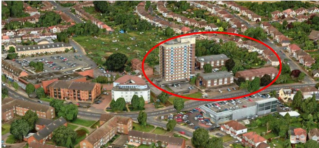
Figure 3: Existing site context (Source: Design & Access statement)
