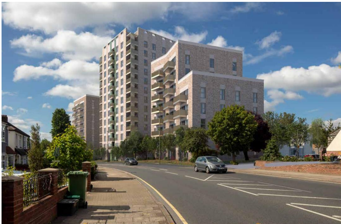
Figure 17: Proposed View from Burnt Ash Lane, outside No.160 (Source: Heritage, Townscape and Visual Impact Assessment (Feb,22))
