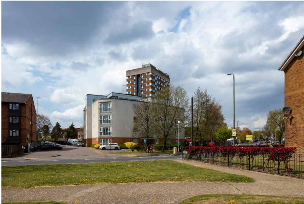
Figure 12: Existing View from Burnt Ash Lane at Ryder Close (Source: Heritage, Townscape and Visual Impact Assessment (Feb, 22))
