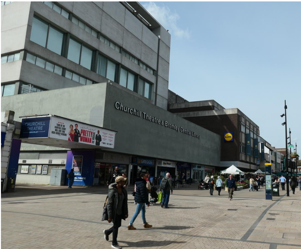
Photo 7: A view of the postwar buildings on the west side of the High Street Character Area, from the south.
