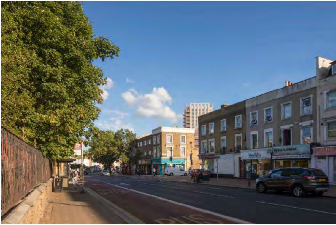
Fig.6.5.1 View 2 - Amended Proposed Development: High Street, adjacent to Watermen's Square (Penge High Street Conservation Area), looking south-east (HTVIA Addendum).
