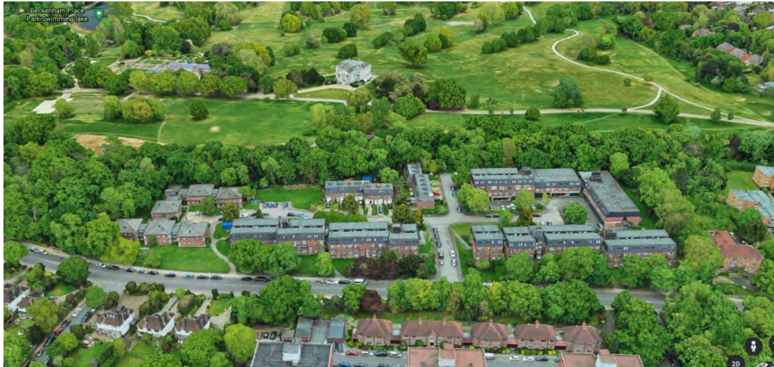
Figure 3: Existing site context (Source: Design & Access statement)
