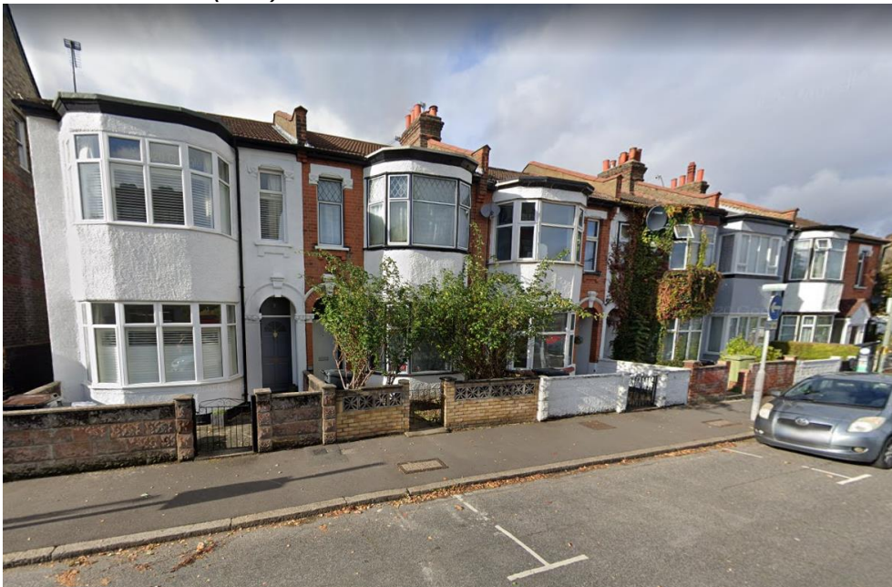
Image 4 - Front elevation of 13-23 Station Road (odds)
