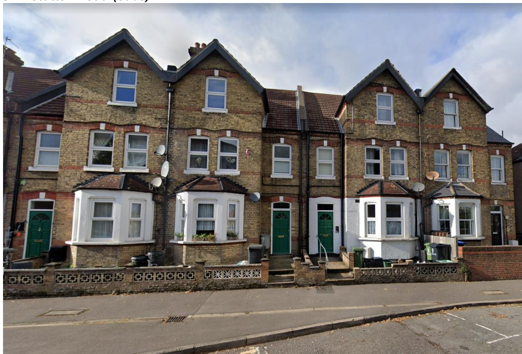
Image 3 - Front elevation of 5-11 Station Road (odds)
