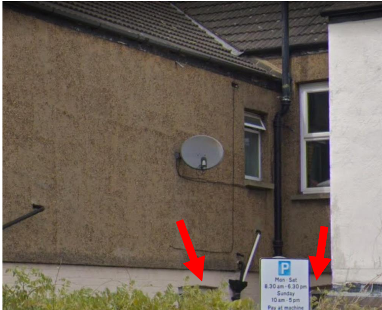
Image 6 - Street view of ground floor windows at no.30
