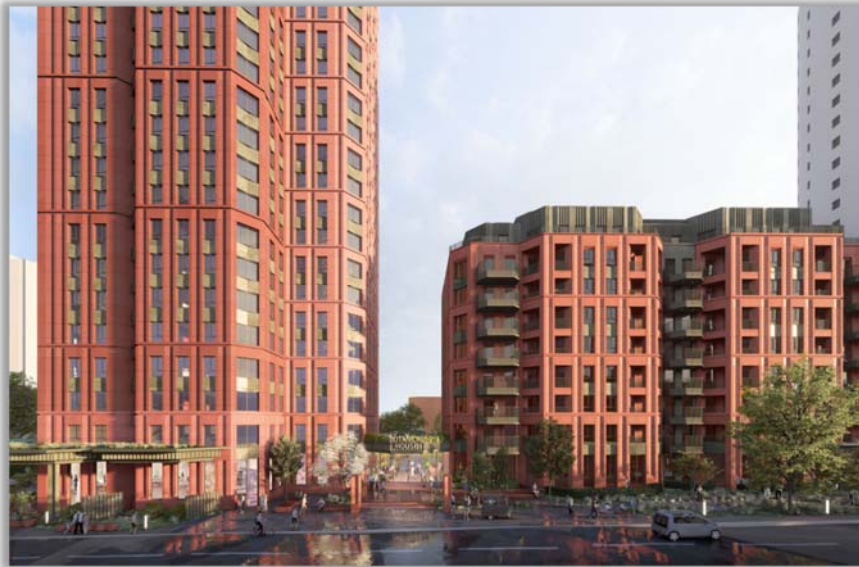
Figure 26: Altyre Road view with the Towers (left) and Mansion Block (right)
