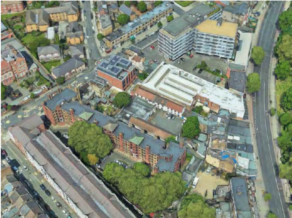
Figure 1: Oblique aerial photograph of the site looking north (Source: Google)
