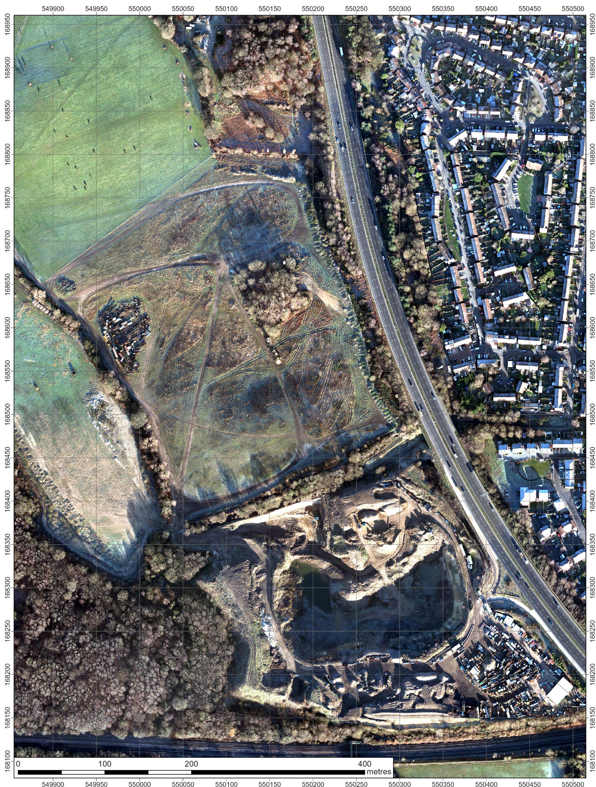
Figure 6 Aerial photography acquired on 6 January 2022 for Land between Bournewood Sand and Gravel Ltd. and Hockenden Lane, Swanley. Image covers the east side of the site
