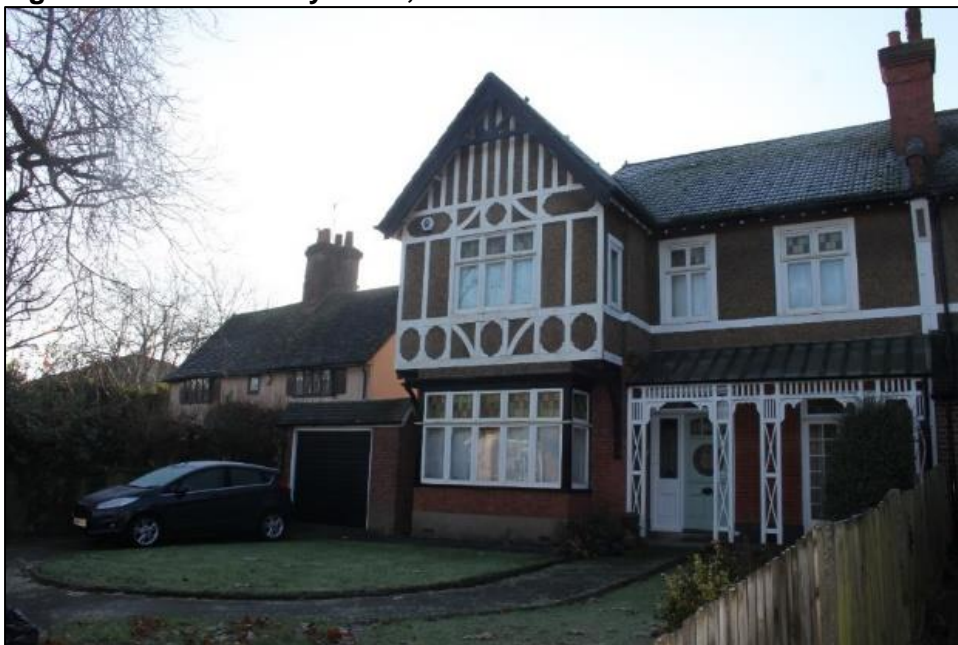
Figure 10: 256 Bromley Road, north east elevation
