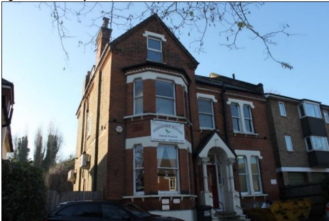
Figure 9: 250 Bromley Road, north east elevation
