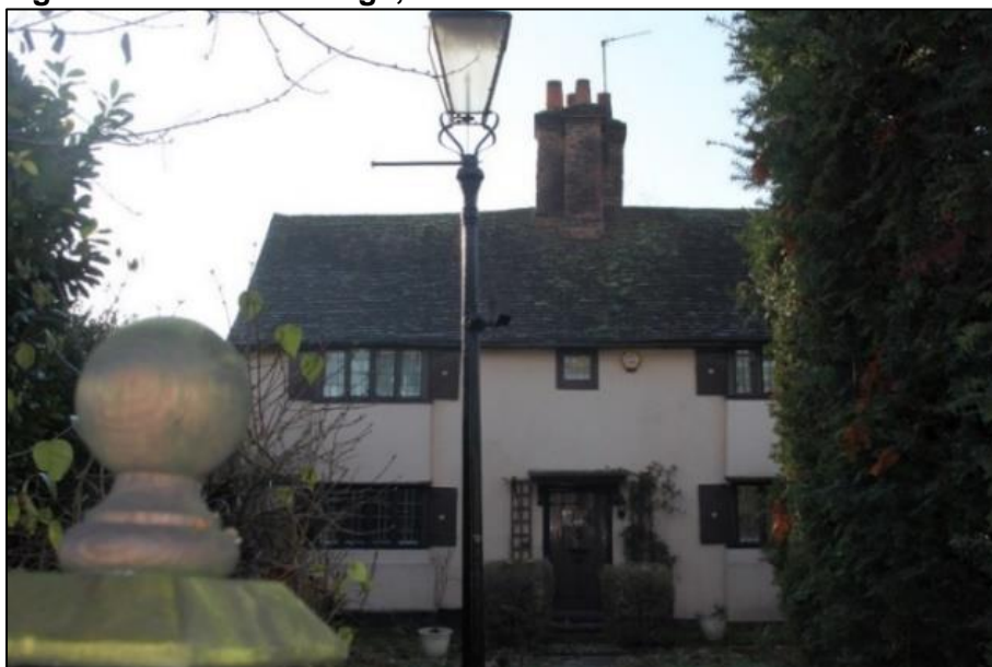
Figure 8: The Old Cottage, north-east elevation
