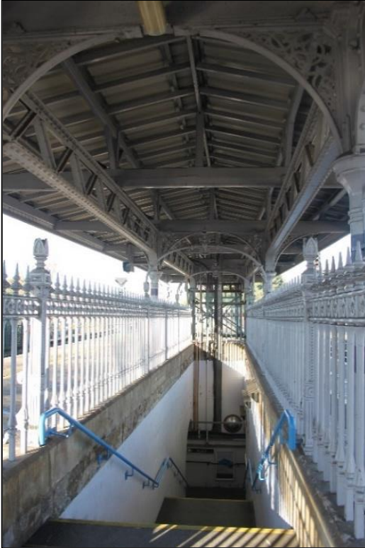
Figure 11: Station platform, ironwork
