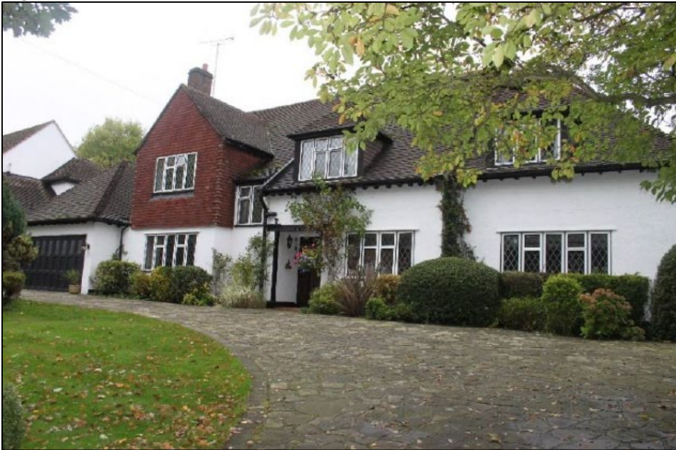
Figure 5: 4 The Covert, south east elevation
