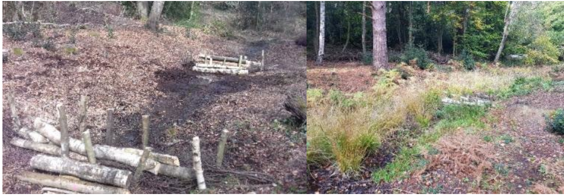
Left: Leaky Dams installed to slow water flow winter 2018, right: the results October 2019
